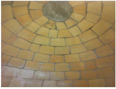
After leaving the sand plug in overnight (even longer for colder conditions) moisture free, Gently knock the bricks out holding the timber template in place. Start with the 2 front and then do the rear. Clean the sand out and any debris and you should be left with the top left picture. You will have to venture inside the oven to clean the internal joints using a DAMP But not wet sponge. Too much water can cause weakness in the mortar.
