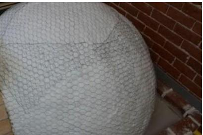
Ceramic insualtion blanket can be irritable And a dust mask an gloves must be worn when handling this product....
