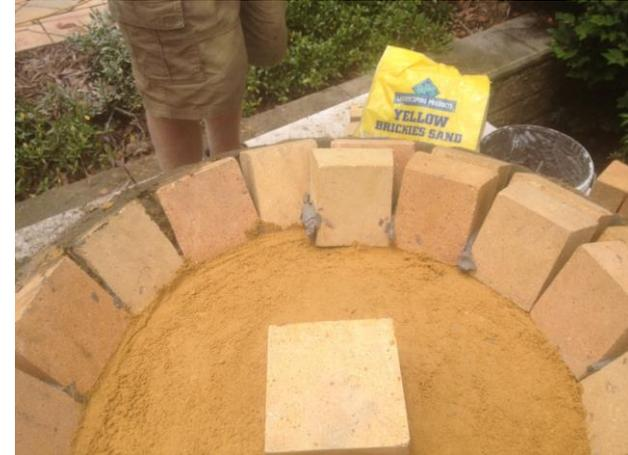
Using the airtset mortar keep doing your 4-5mm internal mortar joints and fondu in between to lock the rear in and strengthen it. Follow the notches on the template for each row
