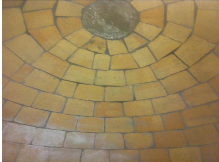
After leaving the sand plug in overnight (even longer for colder conditions) moisture free, Gently knock the bricks out holding the timber template in place. Start with the 2 front and then do the rear. Clean the sand out and any debris and you should be left with the top left picture. You will have to venture inside the oven to clean the internal joints using a DAMP But not wet sponge. Too much water can cause weakness in the mortar.
