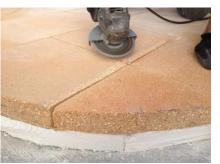
Don't forget to grind and major lips in the floor tiles to save from your pizza peel getting caught and flip them over so the ground edge faces the insulation board
