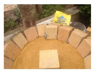
Using the airset mortar keep doing your 4-5mm internal mortar joints and fondu in between to lock the rear in and strengthen it.
