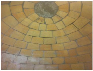
After leaving the sand plug in overnight (even longer for colder conditions) moisture free, Gently knock the bricks out holding the timber template in place. Start with the 2 front and then do the rear.
