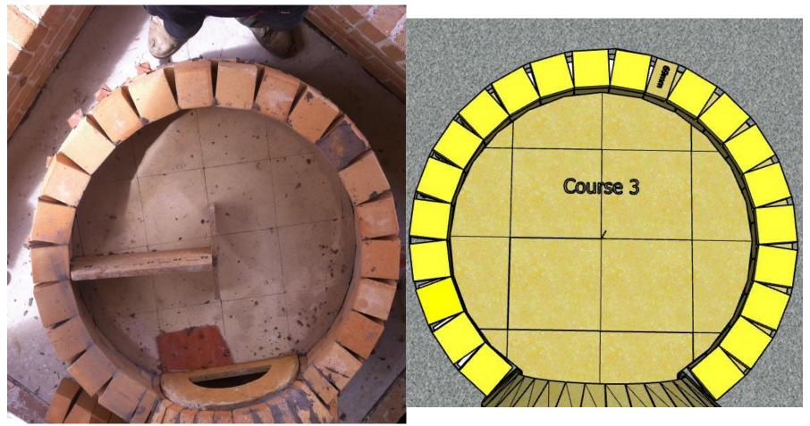
Using the chamber template as a guide from the centre of the oven rotate it around and lay your bricks in the pattern for the second layer Make sure you lean the bricks against the template guide to correctly set the angle
