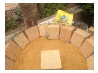
Using the airset mortar keep doing your 4-5mm internal mortar joints and fondu in between to lock the rear in and strengthen it. Follow the notches on the template for each row
