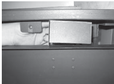
DC Spark Box Bracket Assembly partially removed.
