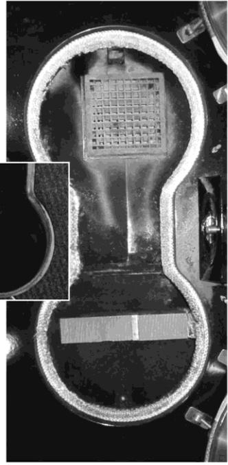
Good draft & clean flue = efficient wood burning, clear flue ways, minimal soot and no tar deposits.
