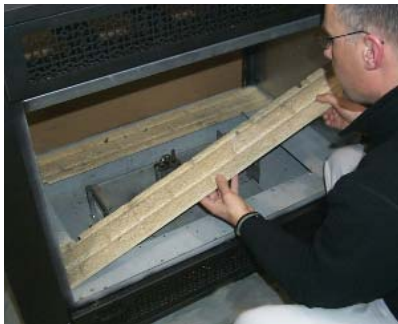
Remove the 2 Long Base Brick Panels
